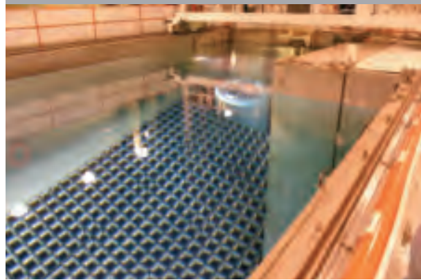
FIGURE 3. WET POOL STORAGE
