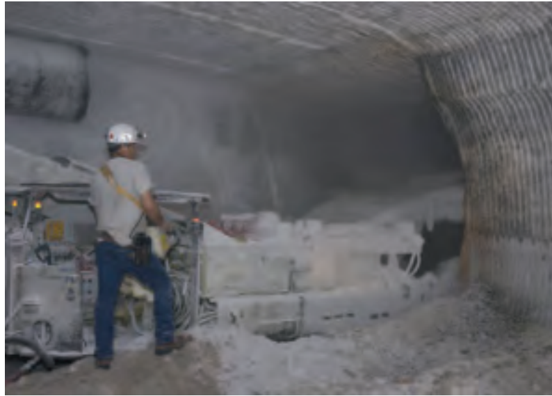
An underground chamber at the WIPP facility.
