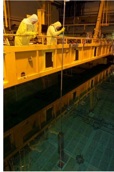
Spent fuel management in the CPP-666 basin
