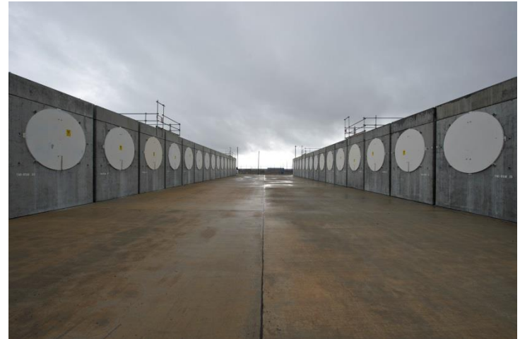
Dry storage of Three Mile Island fuel debris
