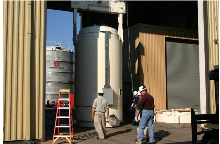
A spent nuclear fuel dry storage cask at the North Anna Nuclear Generating Station in Virginia
