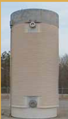
A preferred practice today is to place sufficiently cooled used nuclear fuel in physically robust steel and concrete casks that can be stored either vertically or inserted horizontally into reinforced concrete bunkers.
