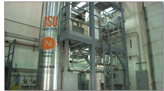
One-third scale Test Facility
