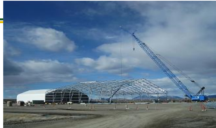
Accelerated Retrieval Project Exhumation Facility construction
