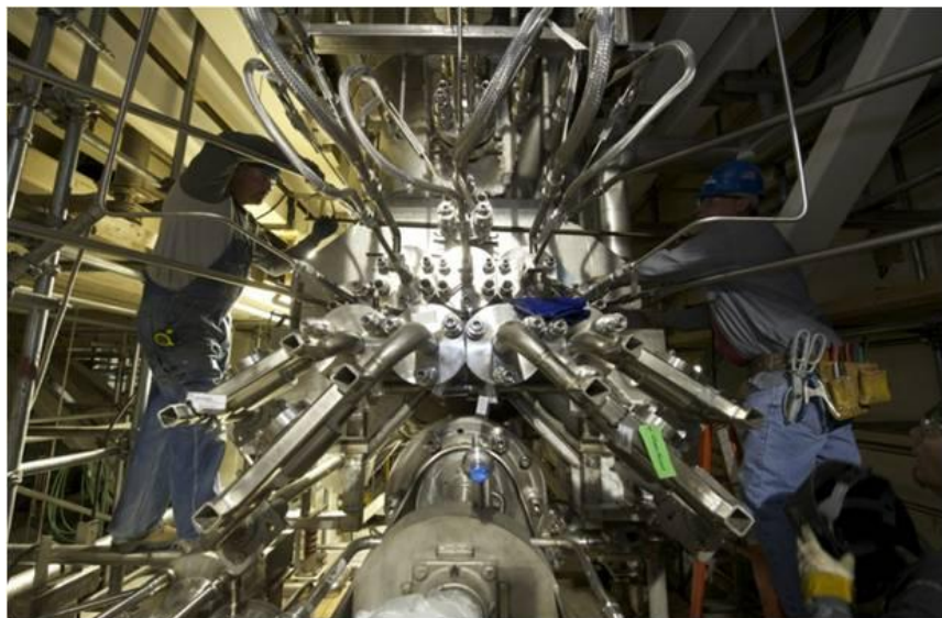
Construction at the IWTU
