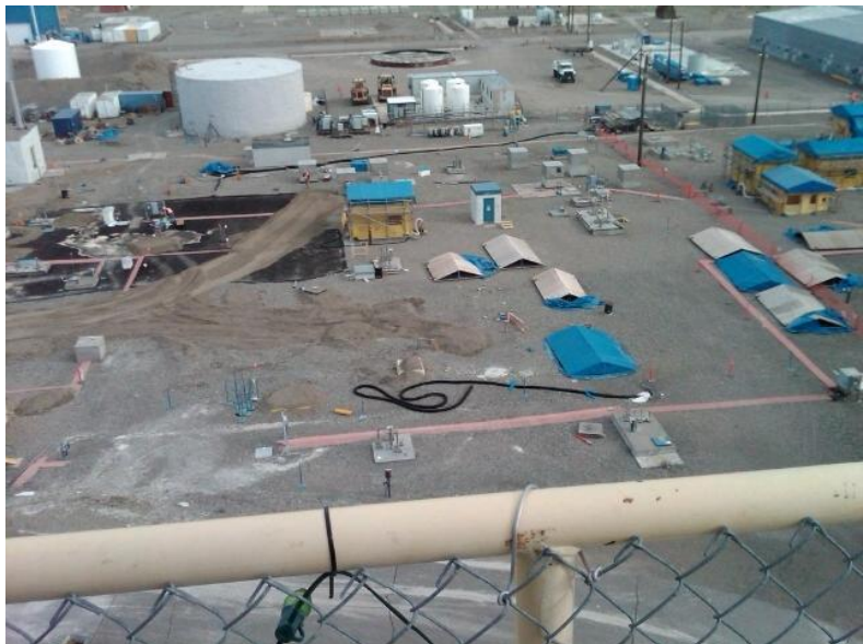
Overhead view of the Tank Farm
