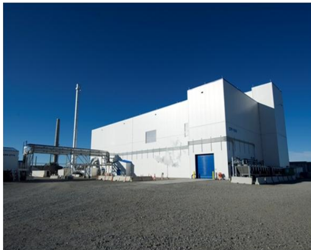
Integrated Waste Treatment Unit
