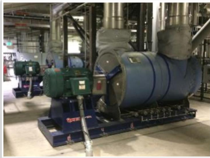
Process Off-Gas Blowers restored
