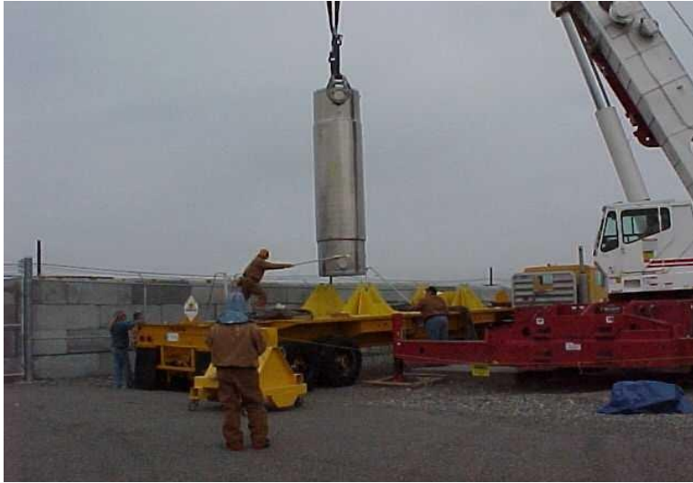
CPP-749 – Positioning cask over truck.
