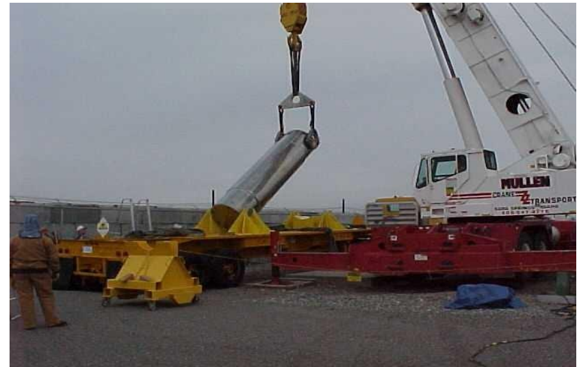
CPP-749 – Laying cask into truck bed.
