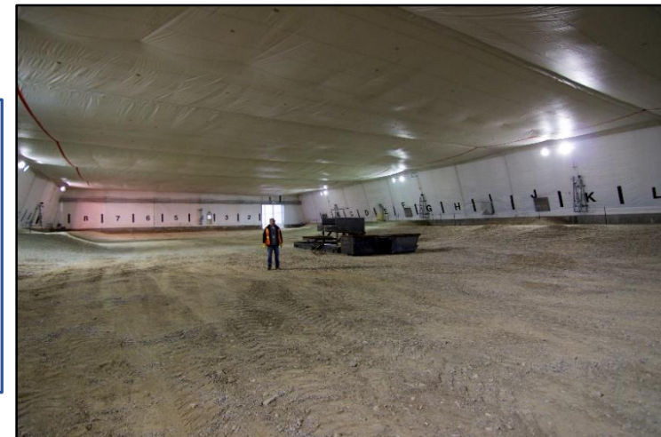
The interior of ARP IX prior to waste exhumation activities.
