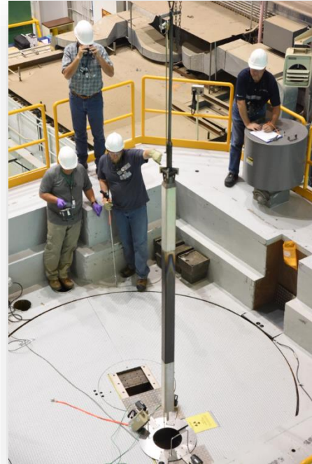
Fuel Assembly Lift from Core
