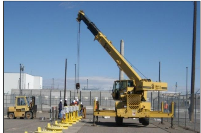
Dry storage at CPP-749
