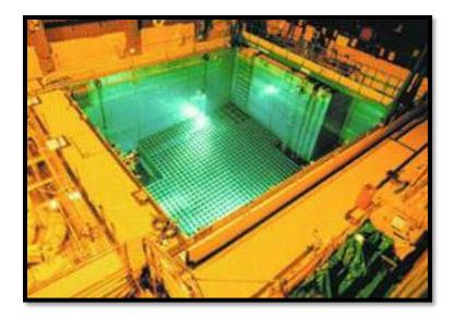
Fig 2. SNF wet storage. Source: [17].
