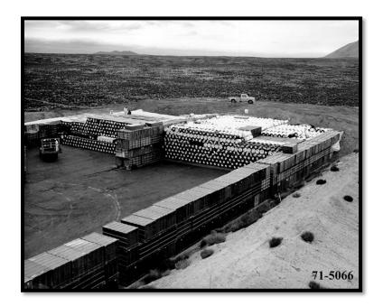
Fig 2. Newly placed drums and boxes of transuranic waste at the RWMC, circa. 1971. The drums and boxes would soon be covered with soil to form a protective berm. *Source:* [6].
