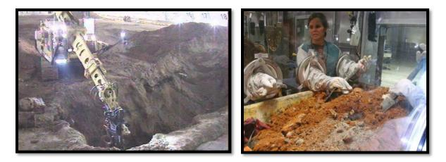
Fig 7. Targeted Waste Exhumation and Inspection Process at ARP. Source: [23]..
