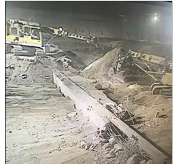
Removal of ARP I&VI foundations within ARP IX
