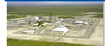
Electro-refining, SNM for Test/R&D
