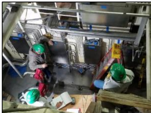
Wet decon control tubing installation inside pipe chase (Pre-COVID)
