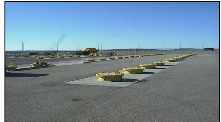
CPP-749, Underground Vault Storage
