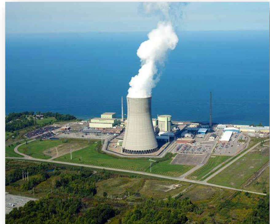
Nine Mile Point (Courtesy of Exelon)
