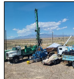
USGS drilling the new ISB treatment well
