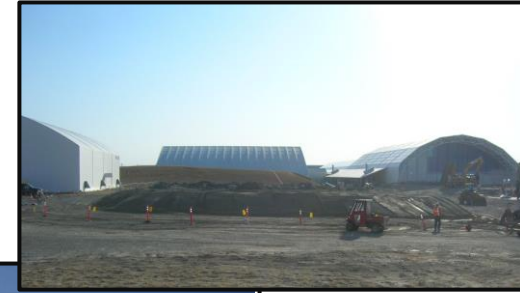
Above: ARP facility dropped and covered in place
