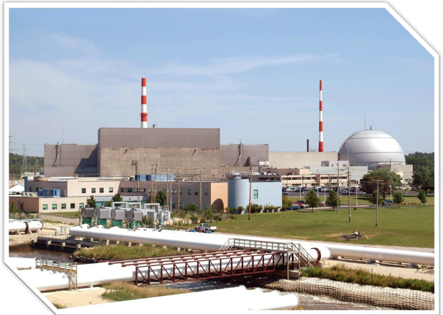
Exelon: Dresden Generating Station
