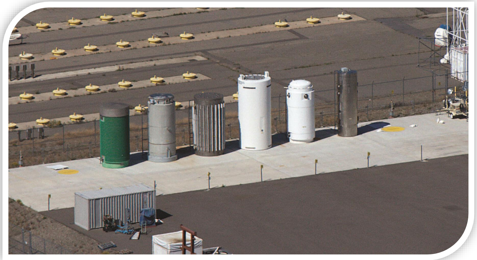
Idaho Nuclear Technology & Engineering Center
