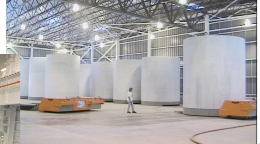
NRF Interim Dry Storage
