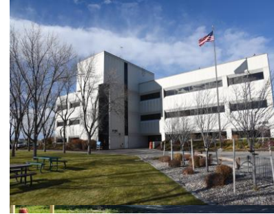
IRC Roof Replacement
