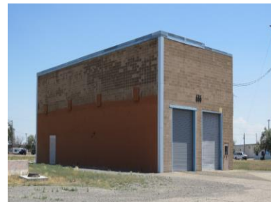
Multi-Program Highbay Upgrades
