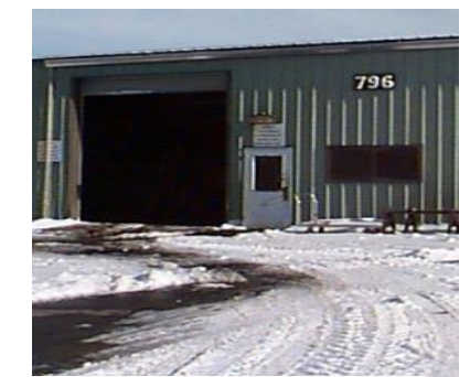
MFC Fabrication Shop Improvements
