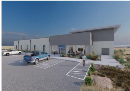
Power Utilities Building
