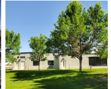
Chemical Storage Facility HVAC Upgrades
