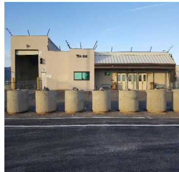
Building 658 Roof Replacement
