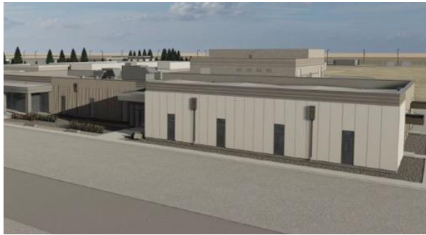
Reactor Support Building
