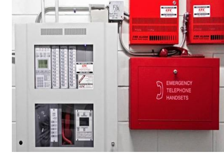
Fire System Upgrades
