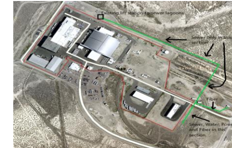
Utility Corridor Upgrade
