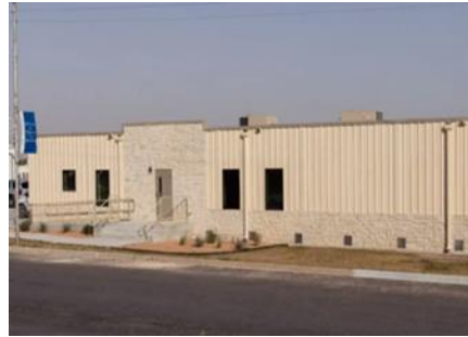
SMC Secure Building at IRC
