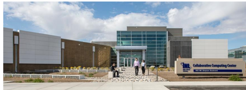
Collaborative Computing Center Cooling Upgrades
