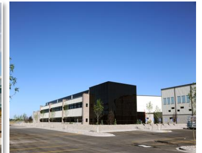
Energy System Laboratory Upgrades
