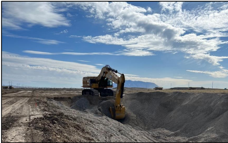
ICDF expansion site preparation
