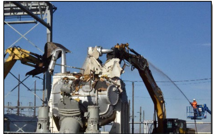
A1W dump condenser dismantlement
