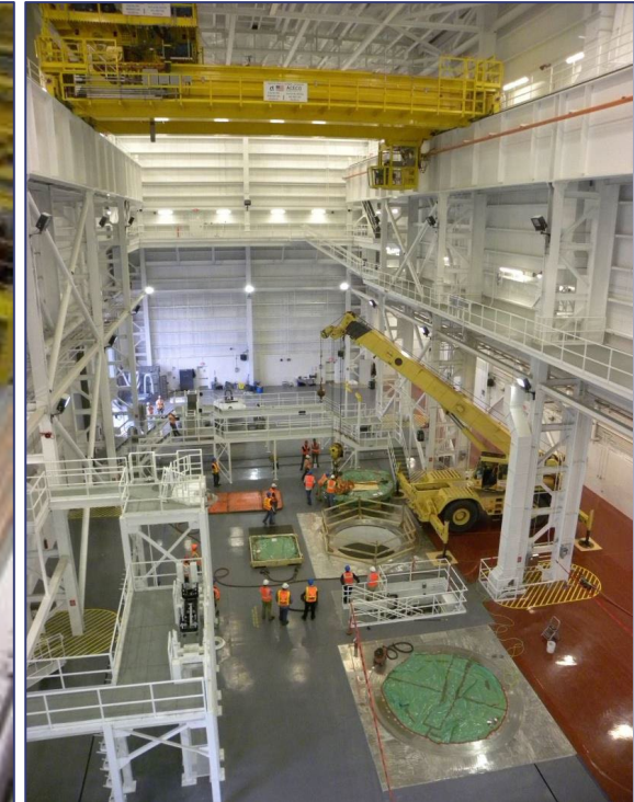
Cask Shipping and Receiving Facility
