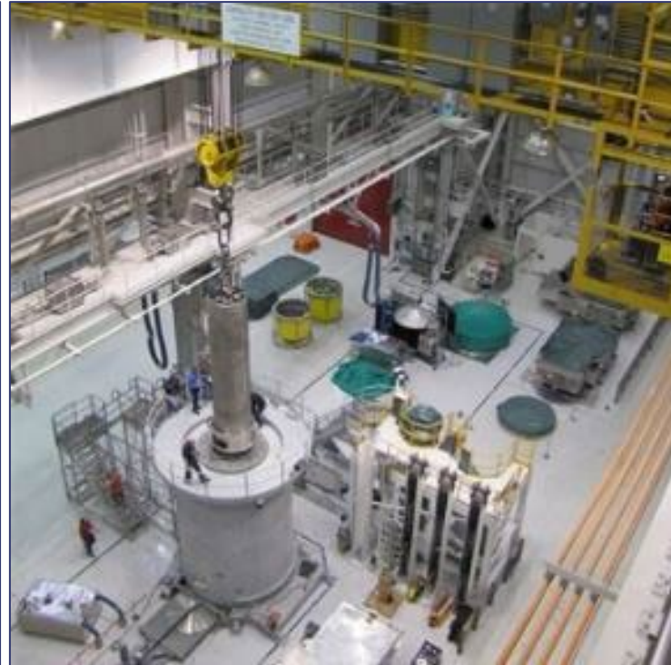
Spent Fuel Packaging Facility
