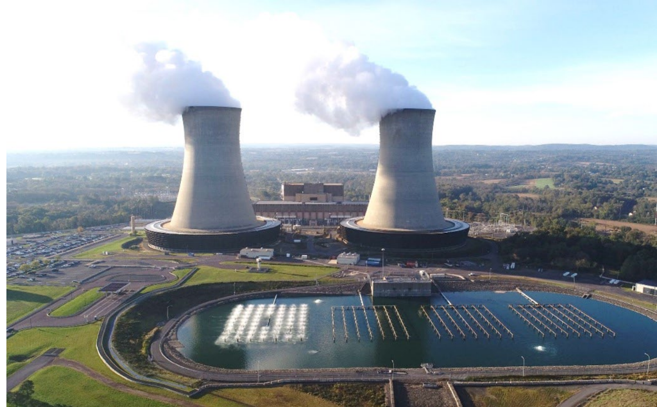
Constellation's Limerick Generating Station in Pottstown, PA
