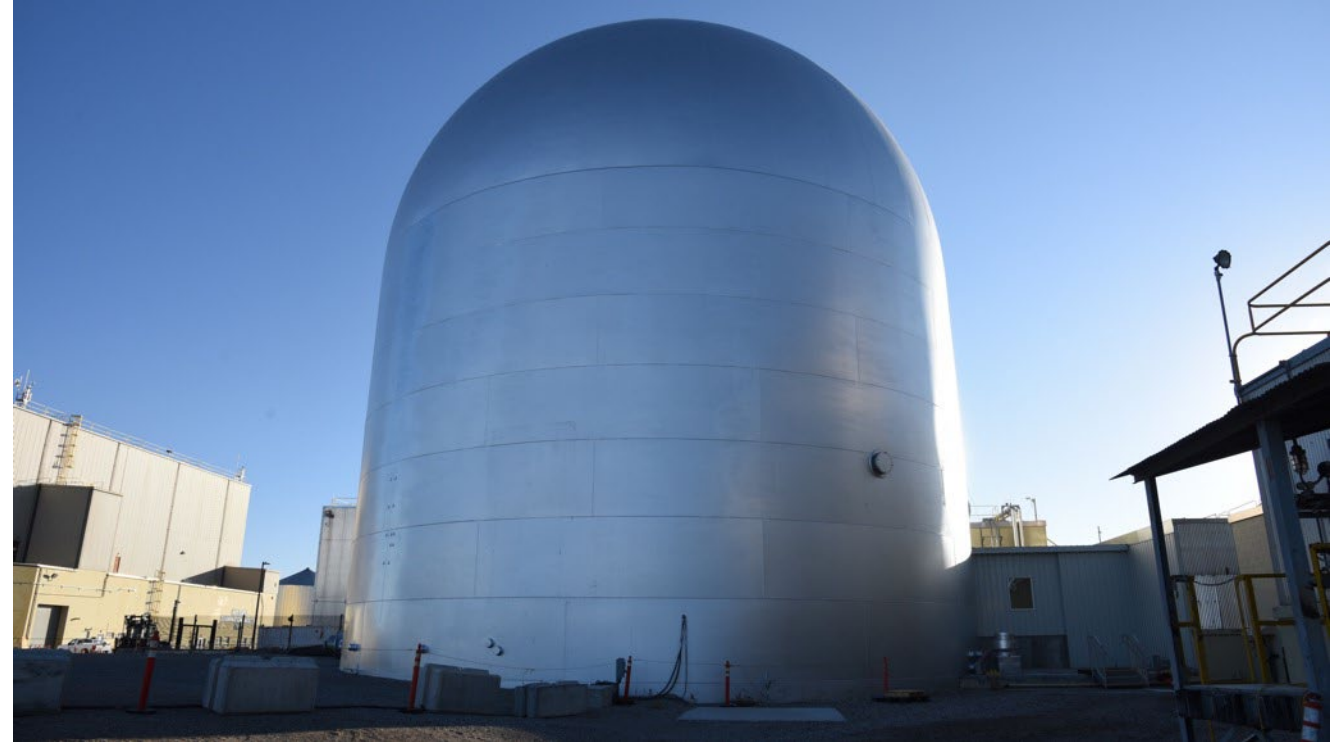
The Experimental Breeder Reactor-II (EBR-II) containment vessel has been used to create the DOME testbed.
