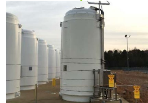
A single storage cask can hold 15 metric ton of uranium (MTU) of commercial spent fuel
