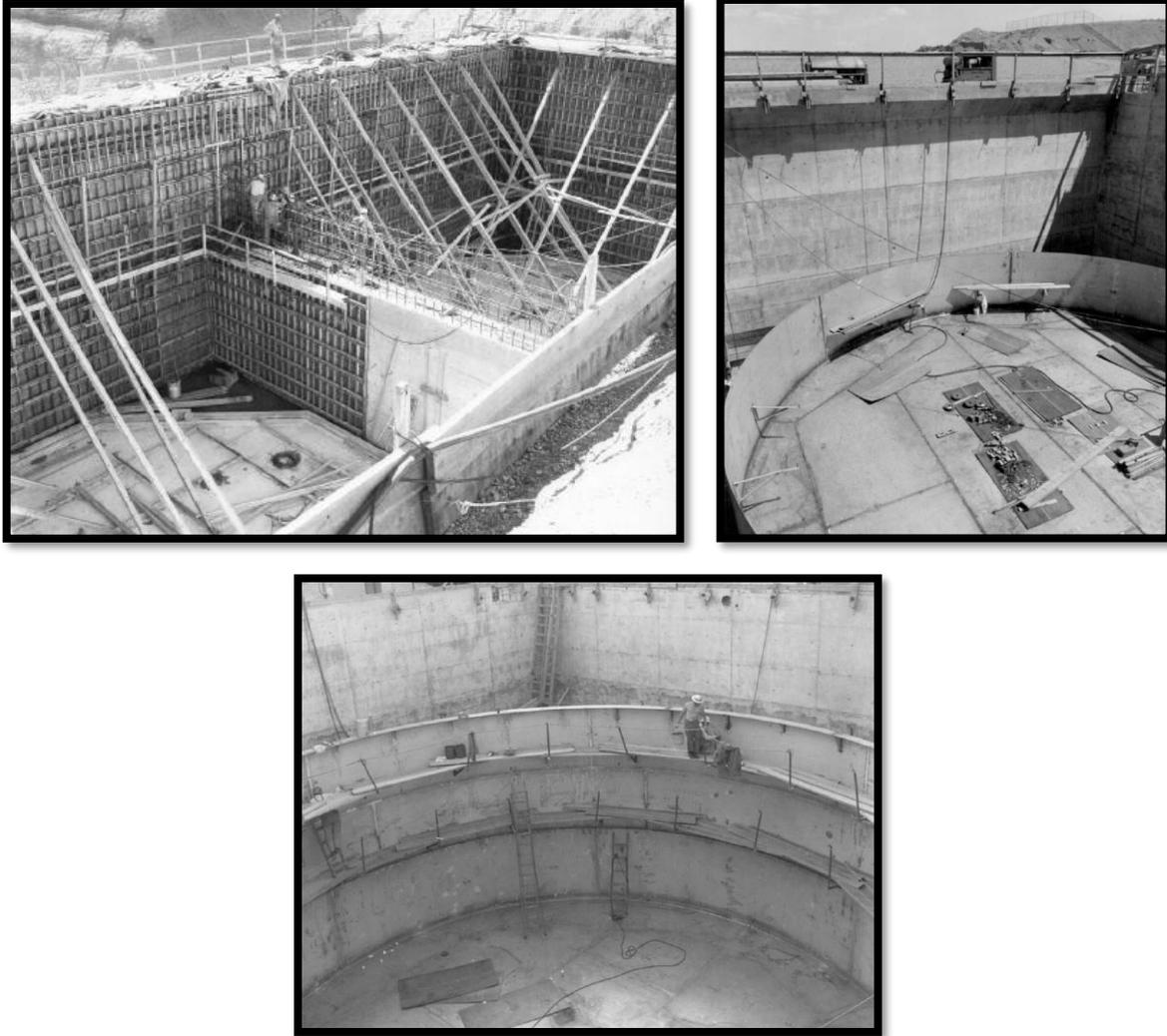
**Fig 3.** Construction of SBW concrete vaults tanks WM-187, WM-188, WM-189, and WM-190.
